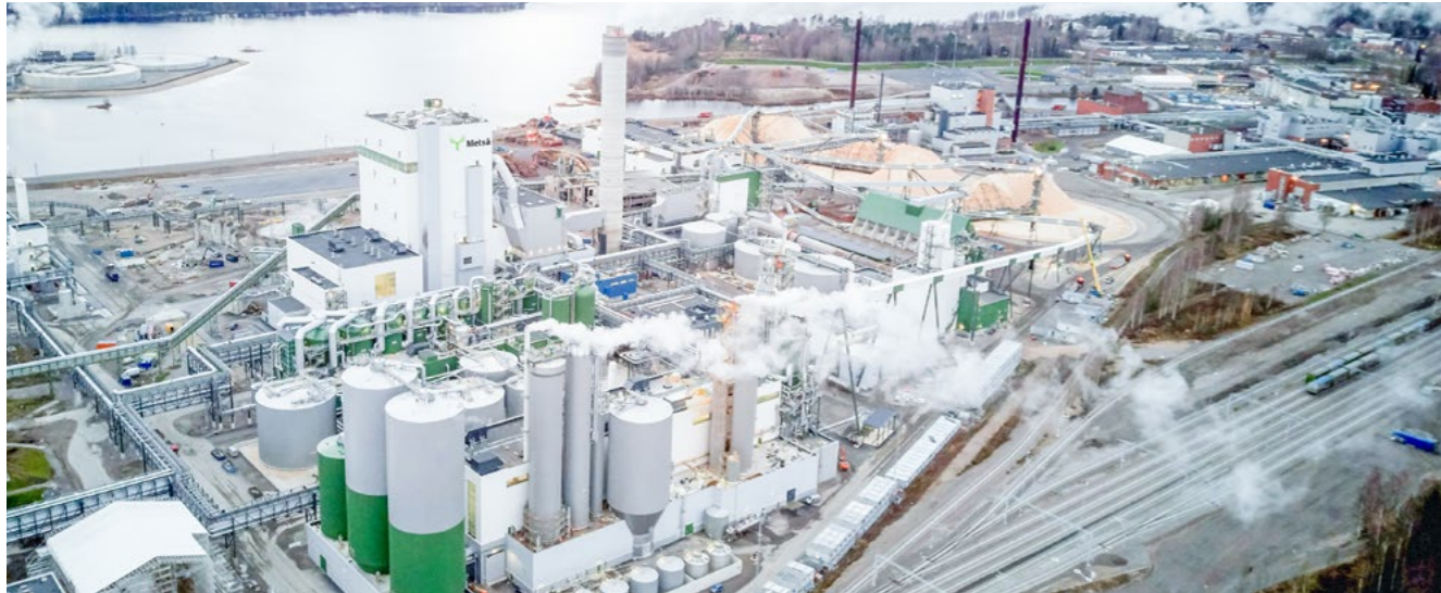
The first installation of a LimeWhite-H filter at Metsä Fibre's Äänekoski bioproduct mill in Finland.
